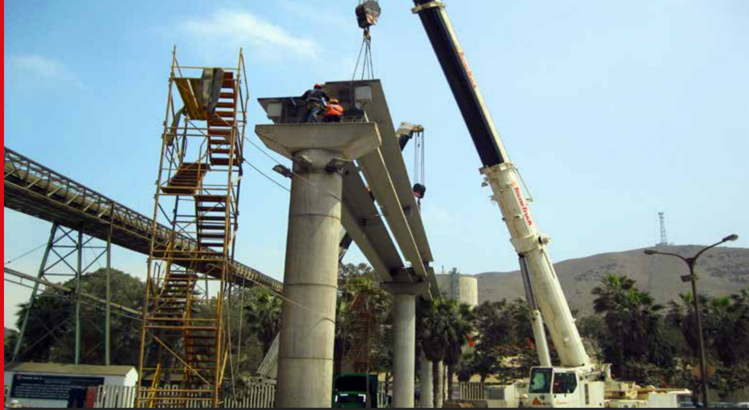
Pipe Rack Cementos Lima
